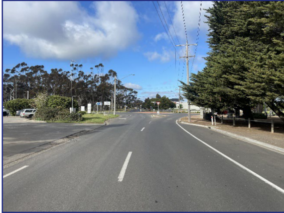
Figure 9: Mill Road - View north-east
