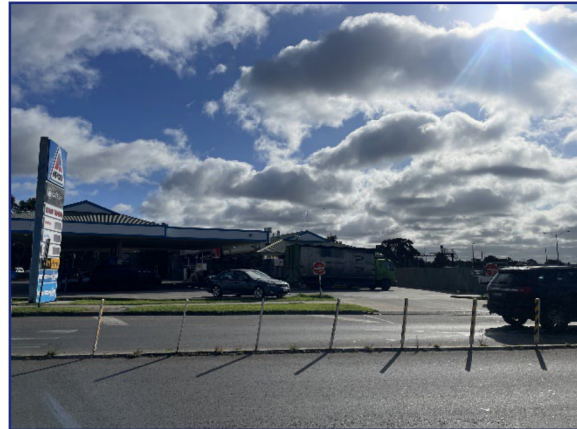
Figure 6: McClelland Avenue – existing eastern crossover
