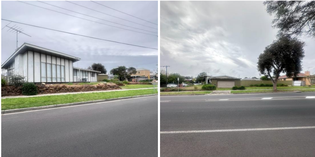
7 Torquay Road as seen from Dorothy Ave (left) and Torquay Road (right)
