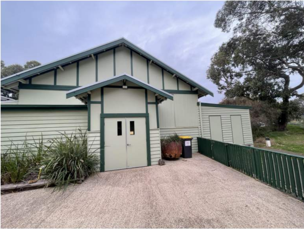
EXISTING REAR VIEW OF BCDC
