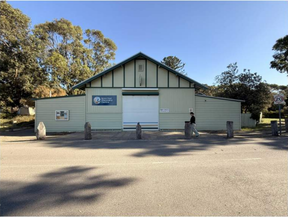
EXISTING VIEW FROM JETTY ROAD
