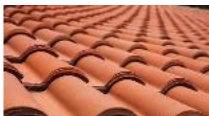
ROOF TERRACOTTA ROOF TILES
