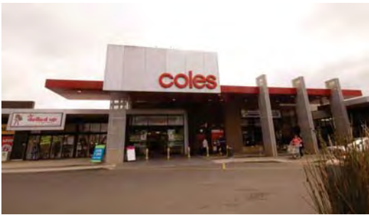
VIEW A EXISTING SHOPPING MALL FRONT
