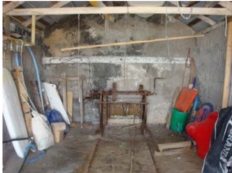
Photo 3.70: Interior, Boat Shed 22 ('Dalhousie'), showing early winch and iron railings. Source: Chris Idle.
