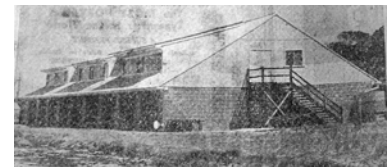
Figure 2.69: Newly-complete Boat Club and Hall Building. Source: Geelong Advertiser , 7 January 1955.
