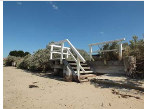
Photo 3.4: Timber access steps to foreshore, Anderson Reserve.
