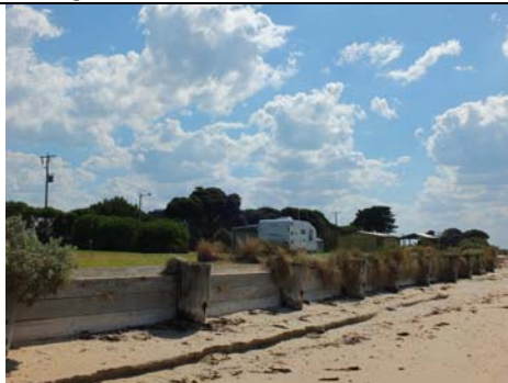
Photo 3.3: Timber sea wall, Anderson Reserve.
