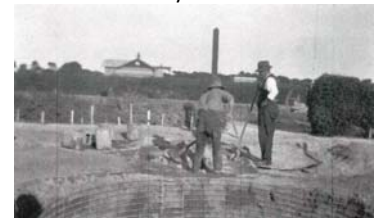
Figure 2.25: W.R. Anderson's "Te Whare" dwelling under construction by H. Lewis, 1920s. Source: Marianne Vessey.
