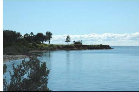
Photo 3.40: View from the south to the Indented Head peninsula, showing erosion of the cliff face.
