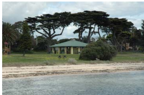
Photo 3.57: Wrathall Memorial Shelter viewed from the jetty.
