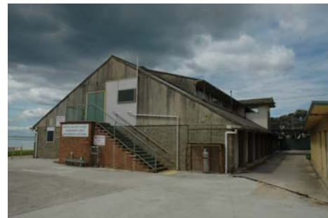
Photo 3.32: Indented Head Boat Club & Hall Building, north elevation.
