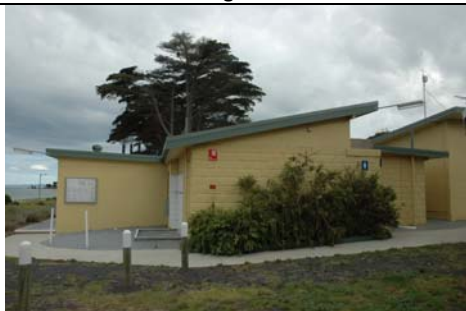
Photo 3.21: North elevation of the altered early amenities block (camp toilets) to the east of the former Administration Building.
