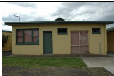
Photo 3.24: South elevation of the former Administration Building.
