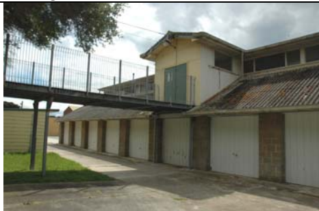
Photo 3.33: Indented Head Boat Club & Hall Building, south elevation, showing first floor entrance portico and walkway bridge.
