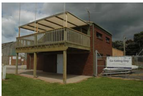
Photo 3.27: Indented Head Yacht Club building, north and east elevations.
