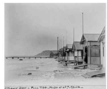
Figure 4.16: Boat Sheds, Barwon Heads, c.1930. Source: Susie Zada collection.
