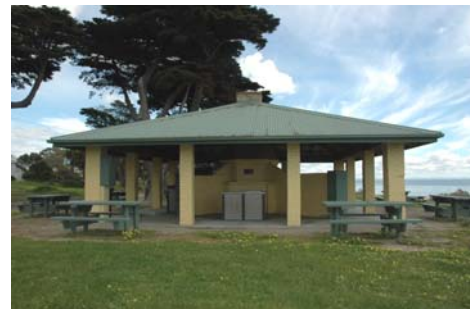
Photo 3.58: South elevation, Wrathall Memorial Shelter.
