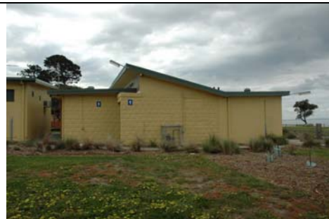
Photo 3.22: South elevation of the altered early amenities block.
