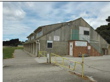
Photo 3.36: Forecourt to the north of the Indented Boat Club & Hall Building.
