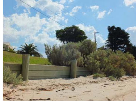
Photo 3.8: Timber sea wall, Aylmer Reserve.
