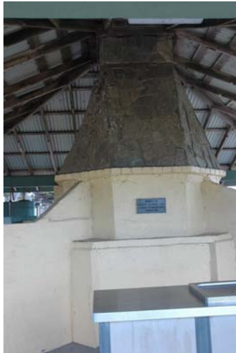
Photo 3.59: Detail of fireplace and flue.
