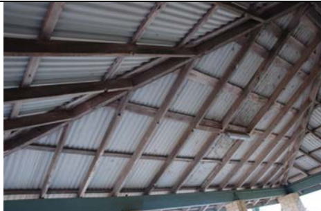
Photo 3.61: Roof structure detail showing recycled timbers.
