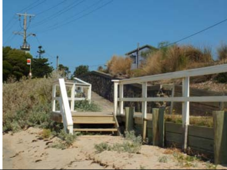
Photo 3.7: Steps, ramp and retaining wall, Aylmer Reserve.
