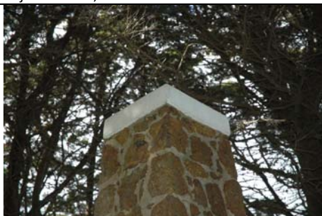
Photo 3.51: Detail of capping of Batman-Flinders Memorial.
