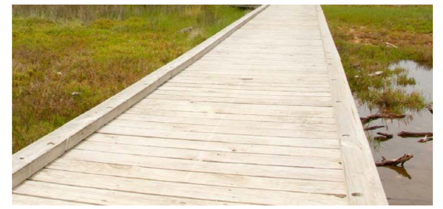
EXAMPLE BOARDWALK IMAGE
