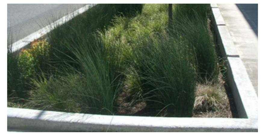
EXAMPLE SWALE TREATMENT BED IMAGE
