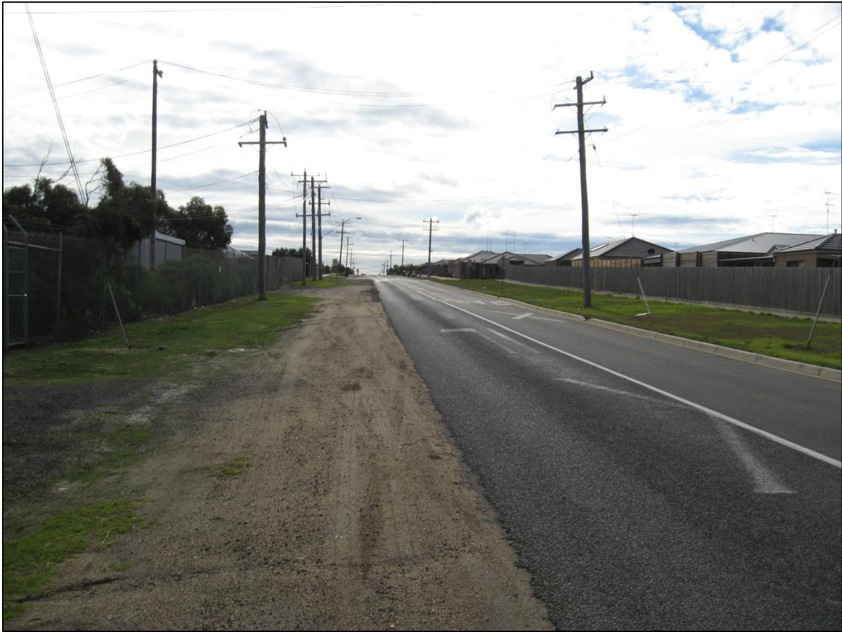
Photo 4 - Ghazeeopore Road, looking north
