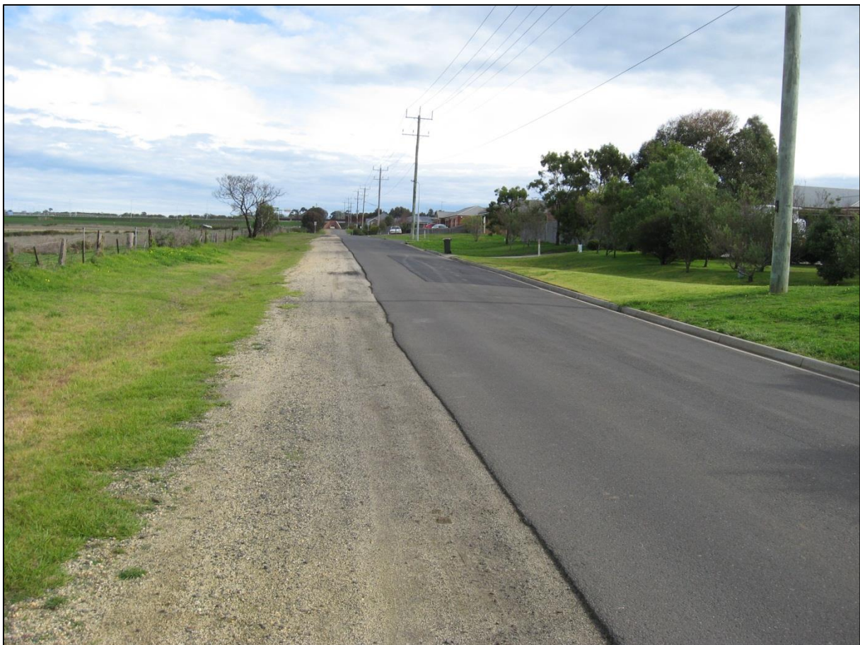
Photo 1 - Hams Road, looking west
