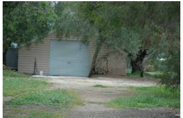
Remnant wall of early outbuilding to the south-west of
