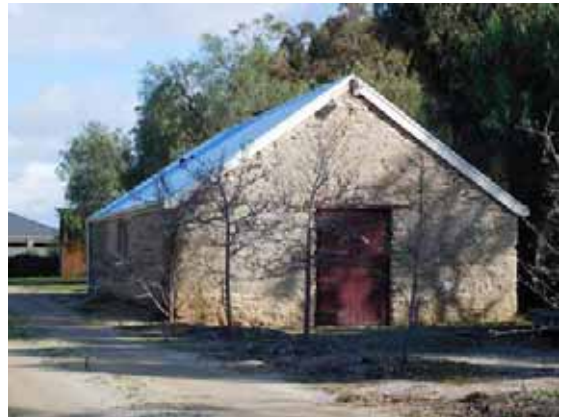
Repaired stables, 2015. Source: David Rowe
