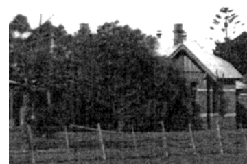
Figure 8.19: Former Inebriates’ Dormitory, Pirra Homestead, 1938-48. Source: Margaret Deller.
