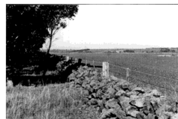
Figure 4.14: Dry Stone Wall, Bacchus Marsh Road, 1998. Source: David Rowe.
