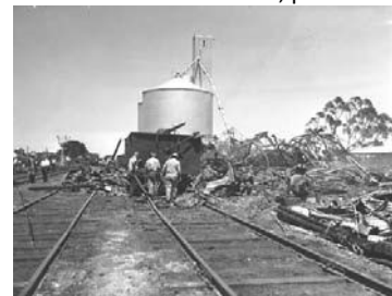
Figure 5.04: Railway officials inspect damaged Chaff Mill Silos after Lara bushfires in 1969. Source: National Library of Australia, accession no. A1200-19.
