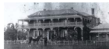
Figure 6.10: Pirra Homestead, c.1910. Source: Geelong Heritage Centre.
