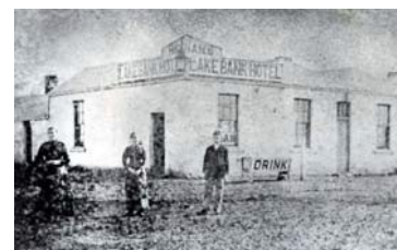
Figure 5.15: Hennan's Lake Bank Hotel, n.d. [c.1884-86]. Source: GRS2009, Geelong Heritage Centre.
