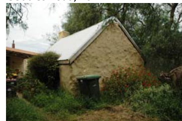
Figure 6.21: Kitchen outbuilding, 80 Gebbies Road, 2012.
