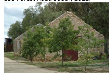
Figure 4.05: Stables remains, Laurence Park, 125 Buckingham Street, 2012.
