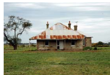
Figure 4.04: Clover Hill Farm House, 155 Forest Road South, 2012.
