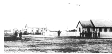
Figure 8.03: View north along Forest Road showing the Wesleyan Methodist Chapel (right) with the Temperance Hall in the background, n.d. Source: Wynd, So Fine a Country , p.160.
