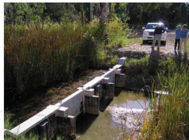
Example of Weir with removable drop boards. For this project our requirements are 1.2m wide weir only. (approx one bay only on the above example).
