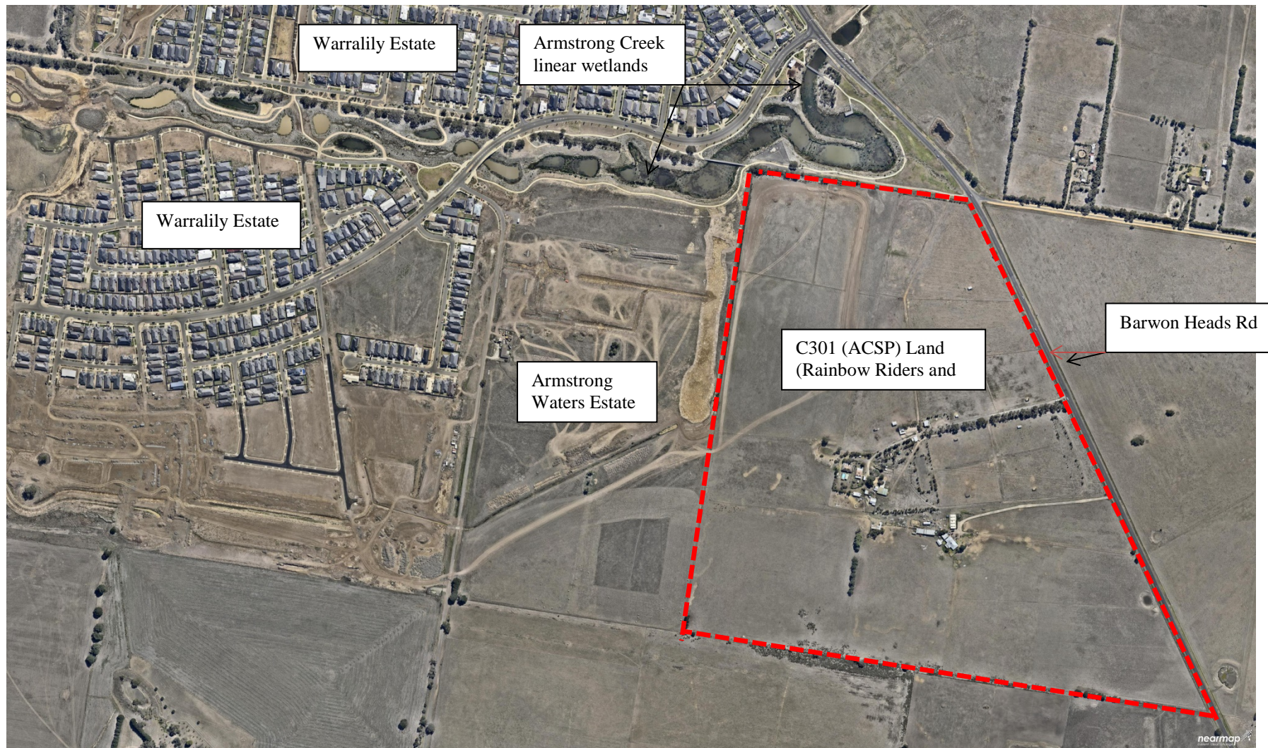
Figure 2 Nearmap.com extract 16 March 2015 showing the C301 land and surrounding development and waterways
