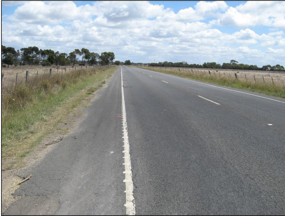
Photo 1: Barwon Heads Road, looking north
