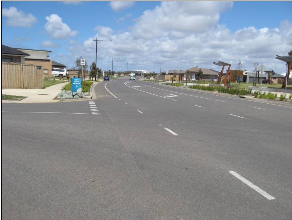
Photo 3: Warralily Boulevard, west approach to Charlemont Road
