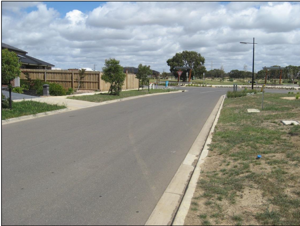
Photo 5: Charlemont Road, looking north
