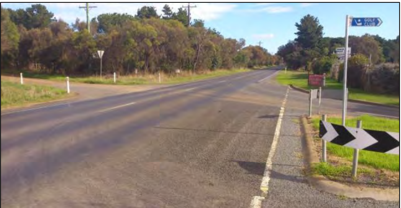
Figure 3-6 Murradoc Road, looking west from Ibbotson Street
