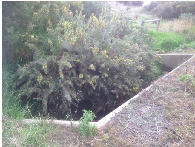
Figure 4.26: Ibbotson Street Culvert Inlet
