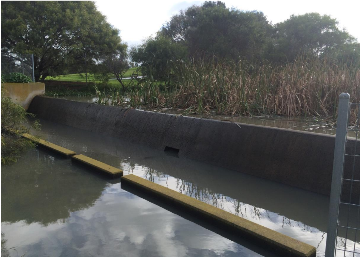
Figure 1.5: St Leonards Lake Weir – Spillway (1.792 m AHD) and Low Flow arrangement
