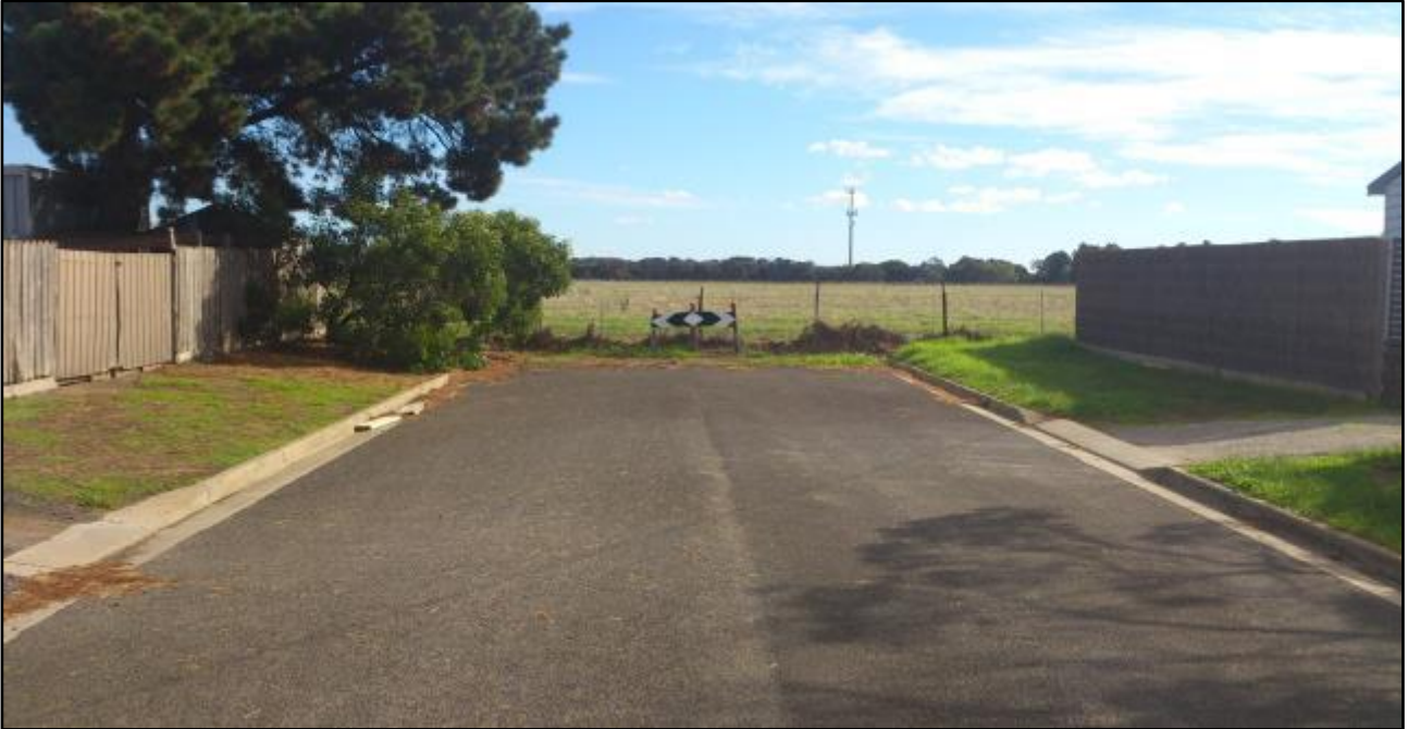
Figure 2-10 Doongara Avenue, looking west from Lake View Crescent
