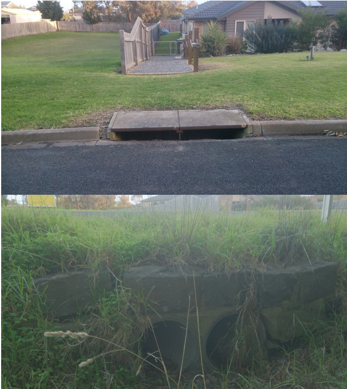
Figure 5 Southern Discharge location – Upstream and Downstream of Bluff Rd
