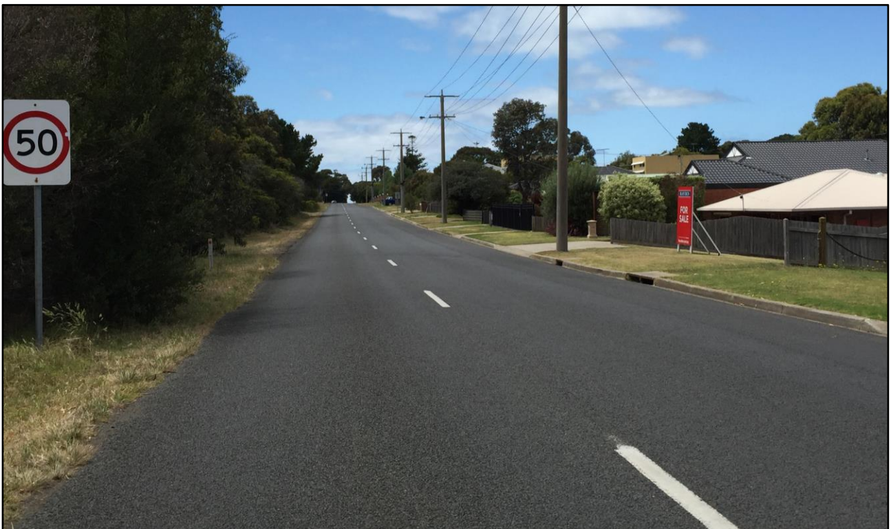
Figure 5-9 Bluff Road, looking east, east of Edwards Point Road
