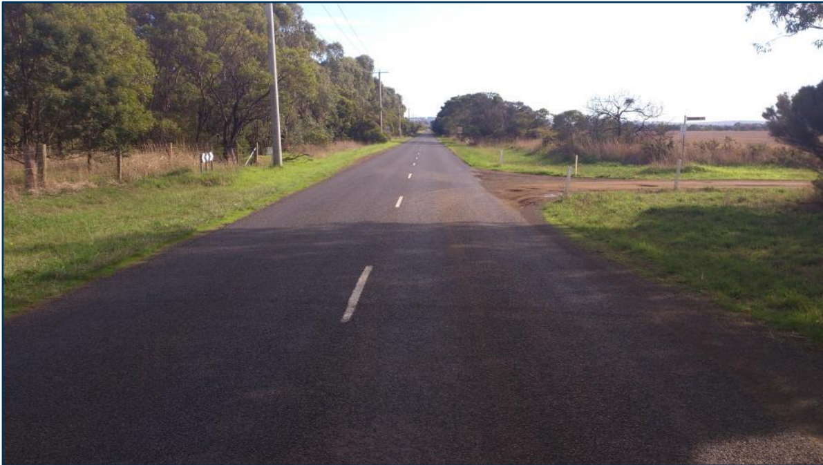
Figure 5-8 Bluff Road, looking west towards Ibbotson Street
