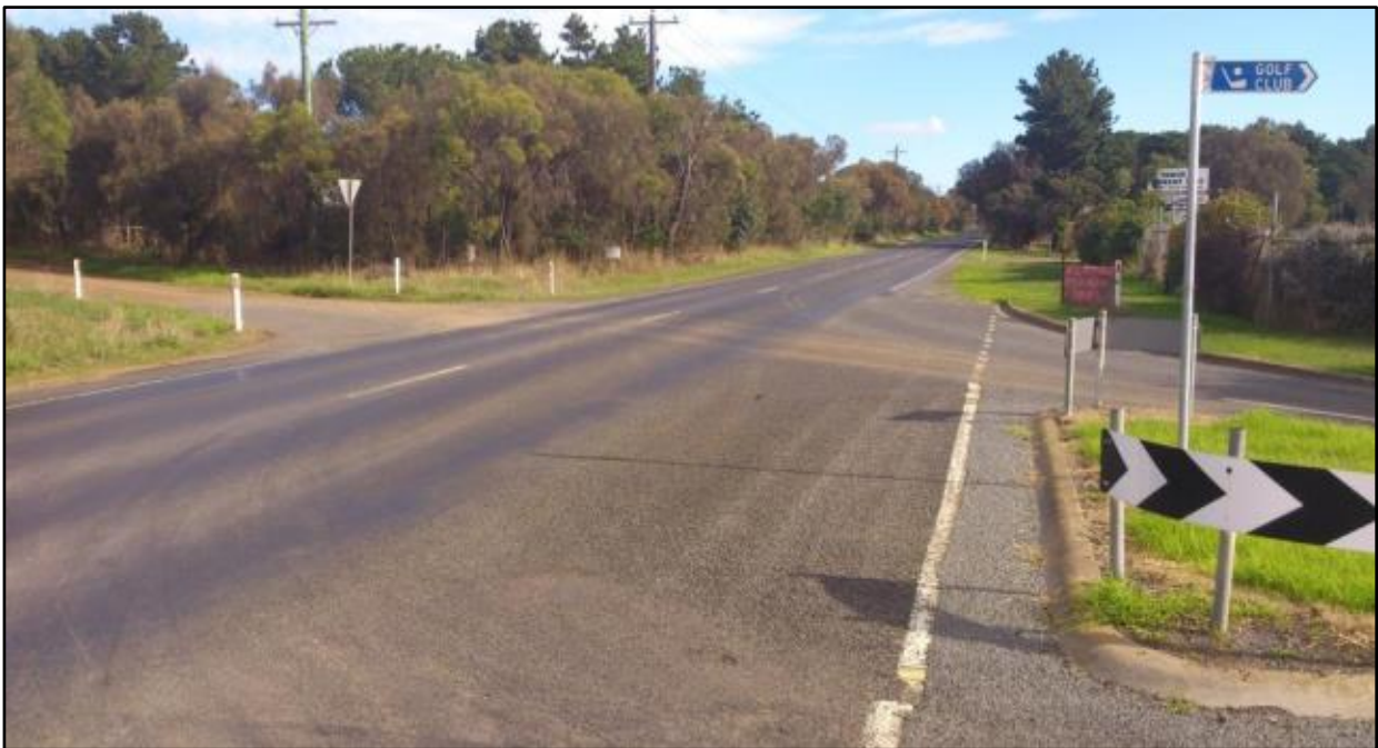
Figure 2-10 Murradoc Road, looking west from Ibbotson Street
