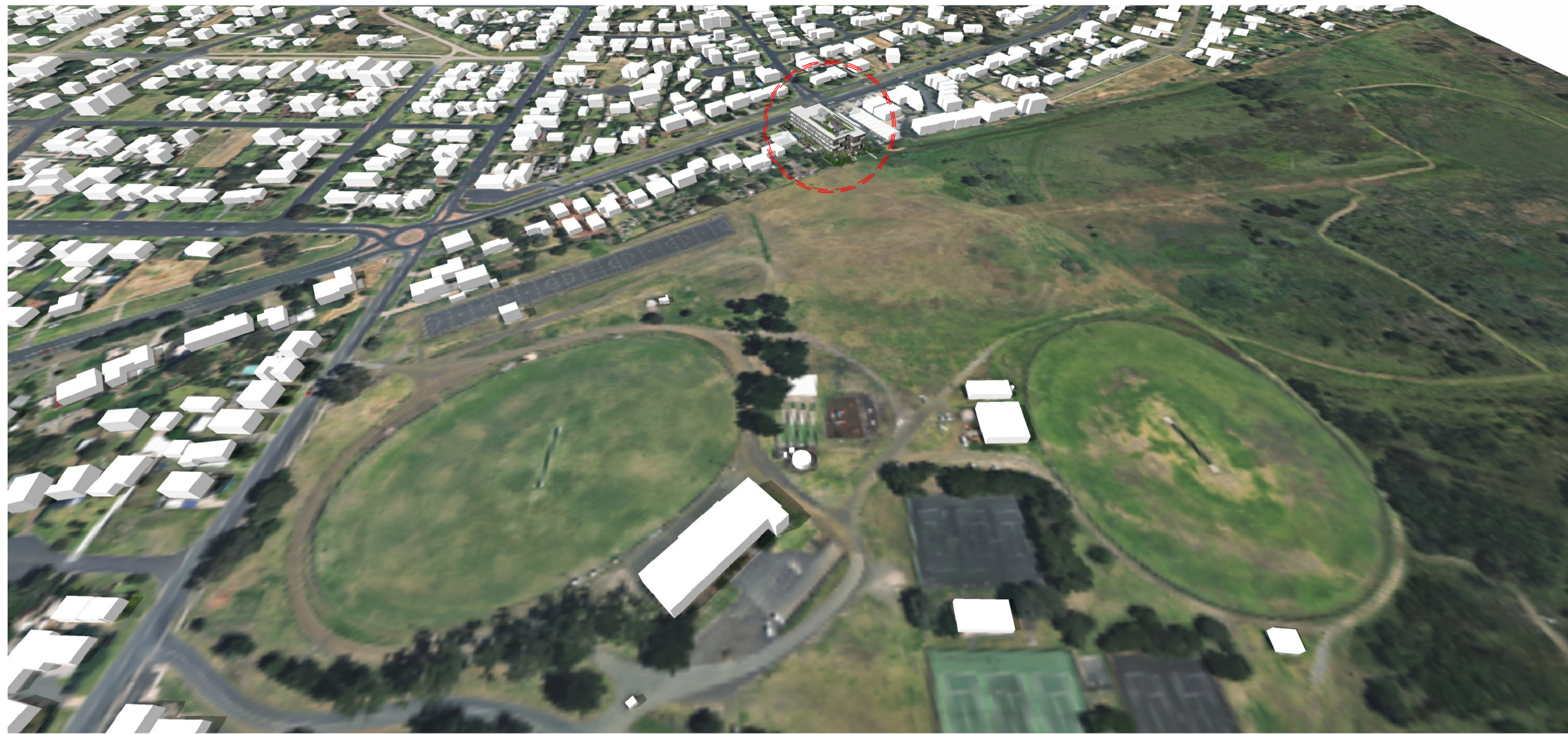
View from Portarlington Recreational Reserve Looking South West
