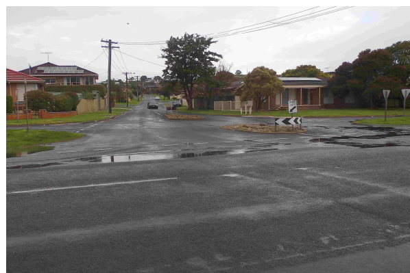
Photo 6: Looking south along Lincoln Drive from Geelong Road.
