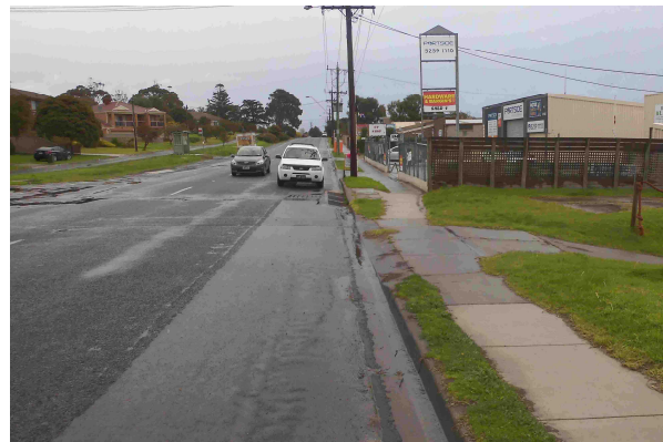
Photo 4: Looking west along the north side of Geelong Road showing footpath.
