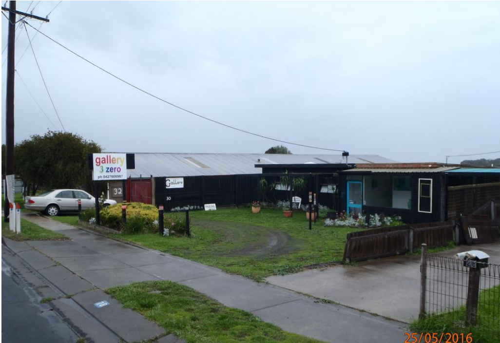
Photo 1 –30 Geelong Rd on right, 32 Geelong Rd (large shed) in centre, looking west.
