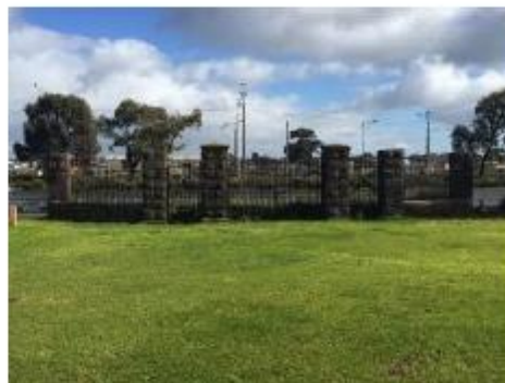
Photo 2: rear view looking west of Osborne House gates, North Geelong, August 2016
