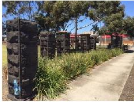
Photo 5: Osborne House bluestone and cast iron gates at Osborne Park, North Geelong Dec 2015
