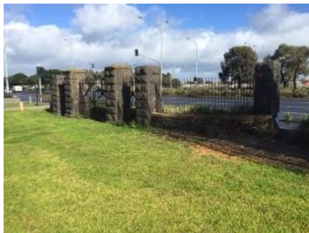
Photo 3: view looking south/west, Osborne Park gates, August 2016
