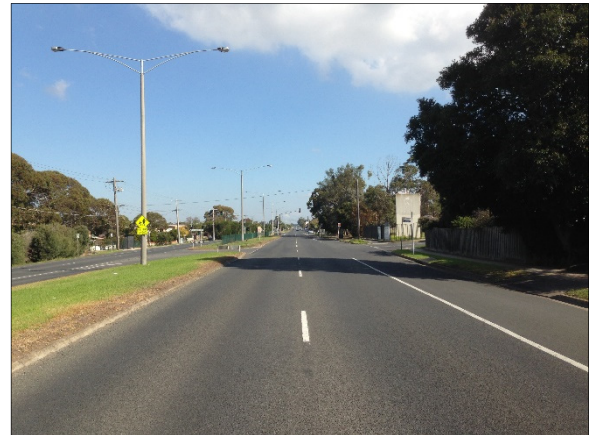
Figure 5: Corio-Waurm Ponds Road – view south-west
