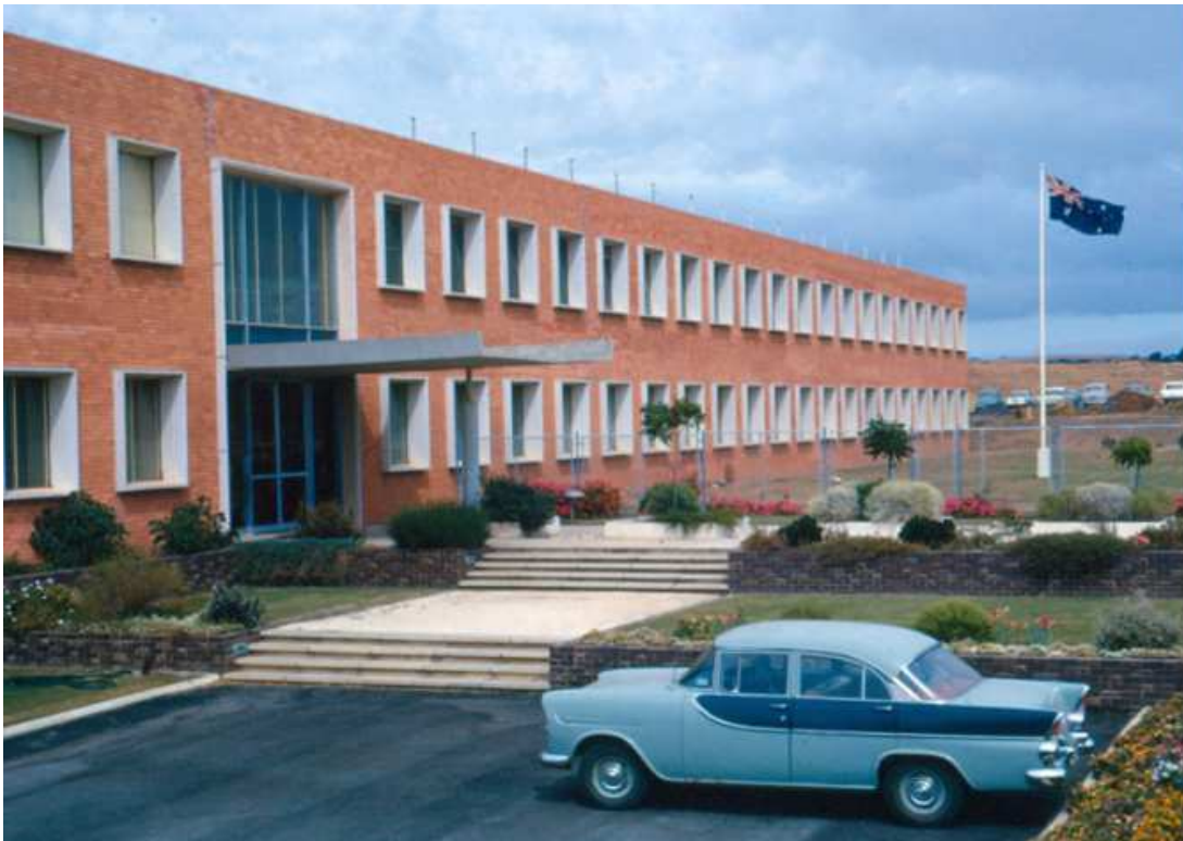
Figure 7 - Exterior view of the Division of Wool Technology
