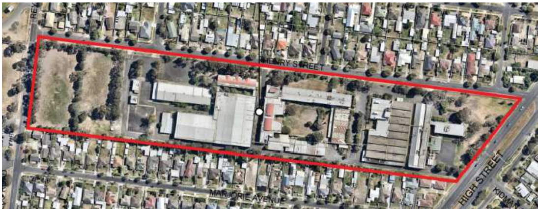
Figure 4 - Aerial Photo prior to demolition
