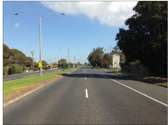
Figure 5: Corio-Waurrn Ponds Road – view south-west
