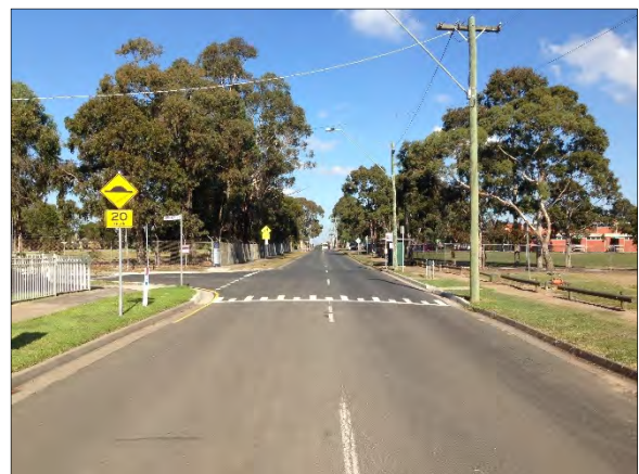
Figure 9: Reynolds Road – view south
