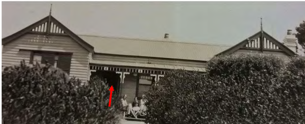
c.1930. The introduced gable end is on the left. The relocated entrance is indicated by an arrow. (Source: Thomas Family)
