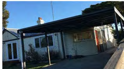
Rear of the house
