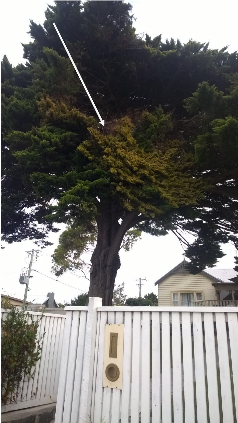
View of the tree from Bridge Street in early January 2017. The arrowed branch with the yellow foliage has recently fractured.
