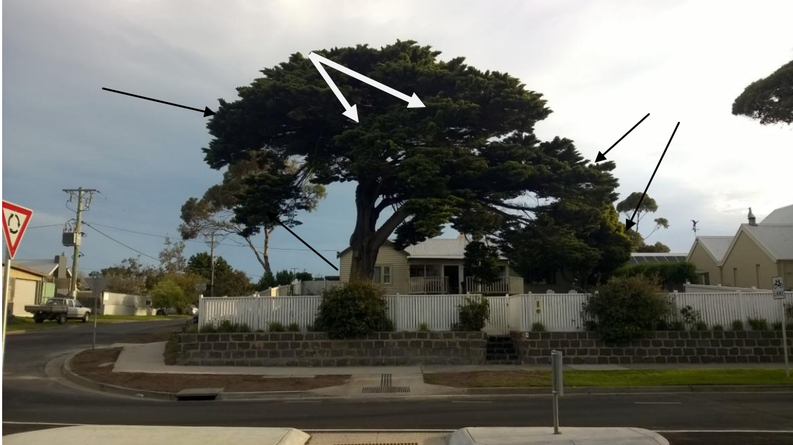
View of the tree looking south in October 2016 with the recently fracture branch arrowed in white. Other high risk boughs are arrowed in black.
