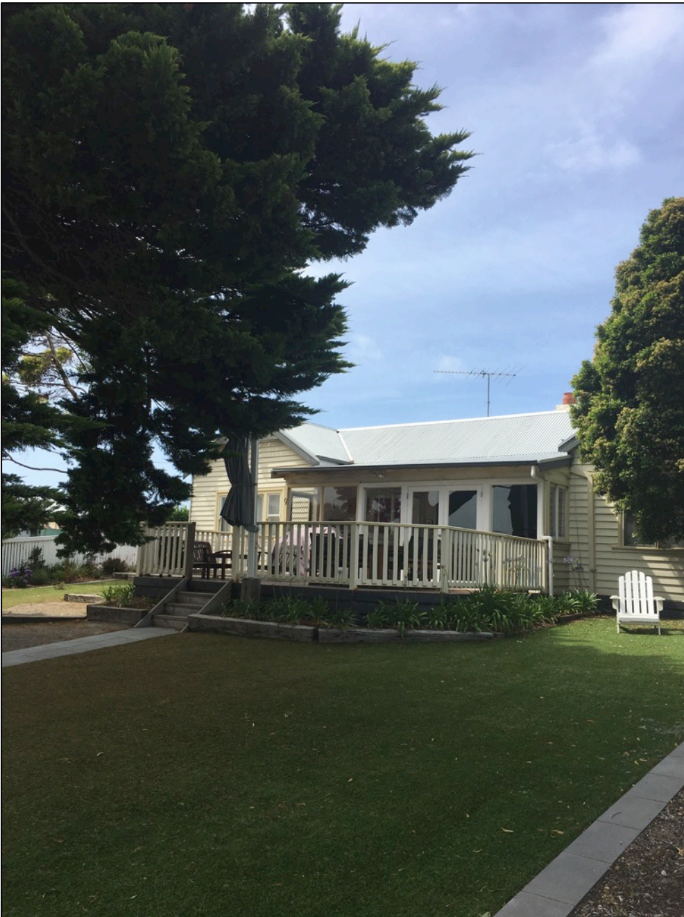
Figure 10: Subject site from driveway of adjoining property – (11 Bridge Road) (GJM Heritage, 14 December 2016)
