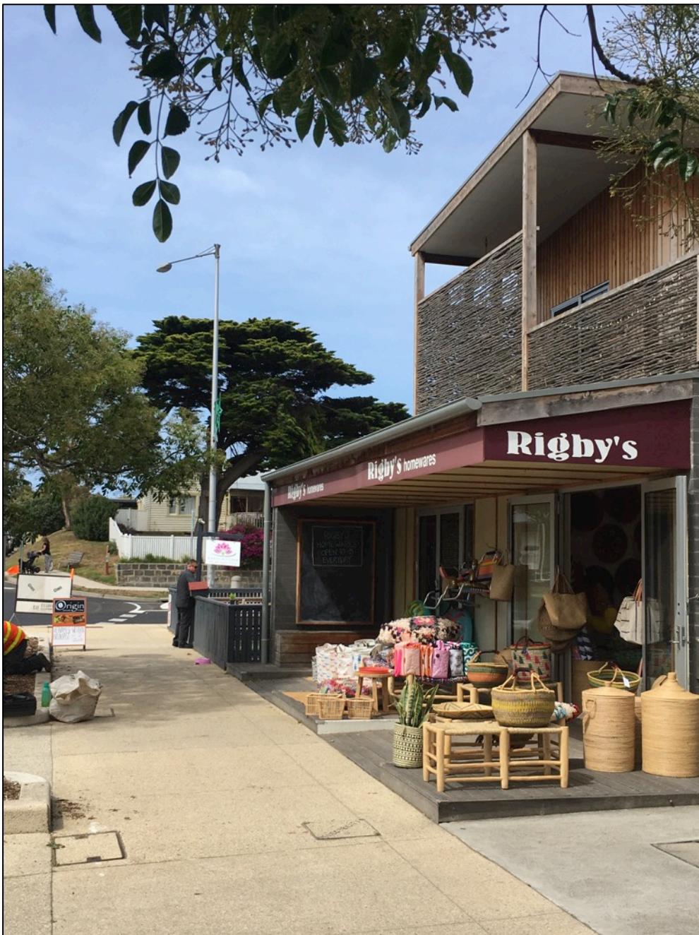
Figure 11: Subject site – viewed from western side of Hitchcock Avenue (GJM Heritage, 14 December 2016)
