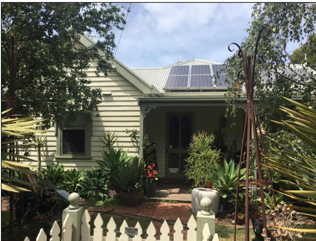
Figure 15: 31 Ozone Road, Barwon Heads (GJM Heritage, 14 December 2016)
