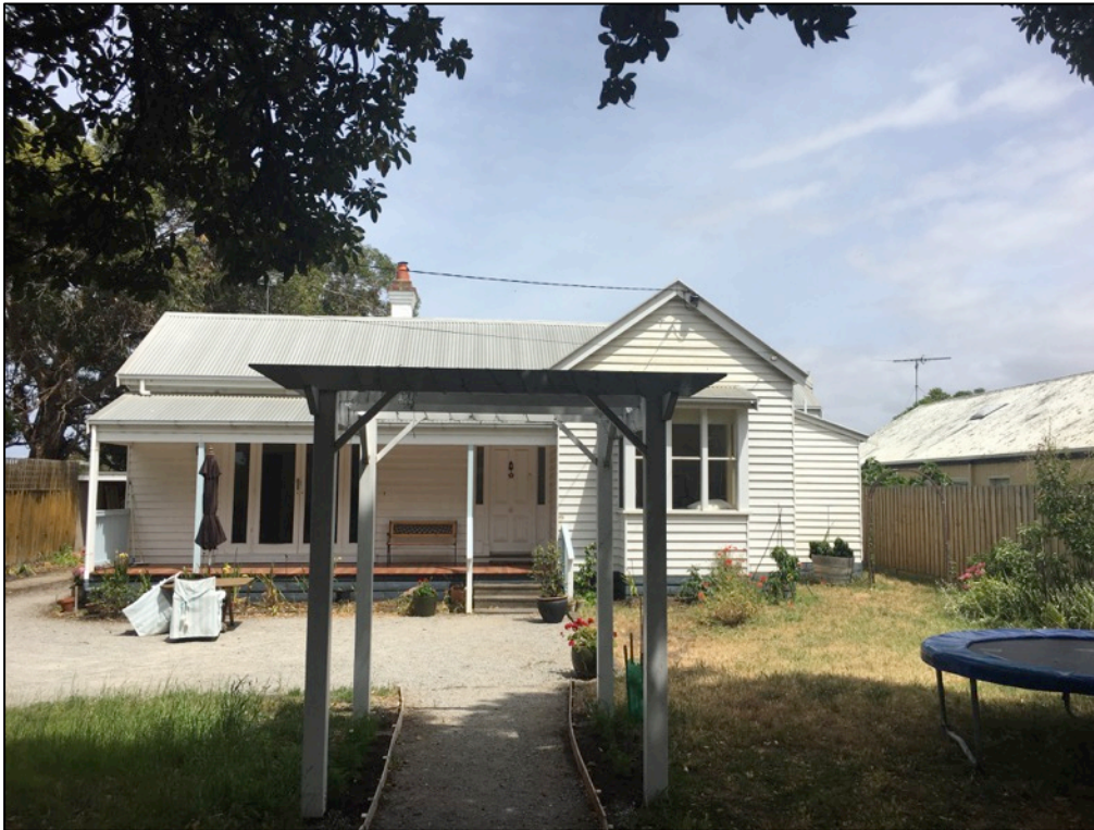
Figure 16: 29 Seaview Avenue, Barwon Heads (GJM Heritage, 14 December 2016)
