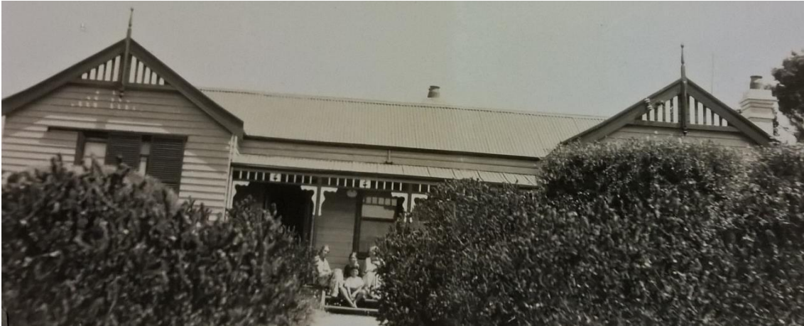
Figure 6 Photograph of house following addition of south gable-ended wing and alterations to verandah, c. 1930s Source: Heritage Values Review , RBA Architects & Conservation Consultants
