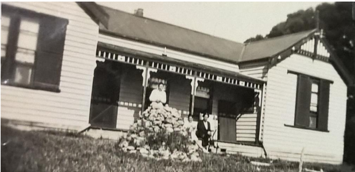
Figure 7 Photograph of 9 Bridge Road following modifications; note new gable-ended wing and alterations to windows and verandah, c. 1930s Source: Heritage Values Review , RBA Architects & Conservation Consultants
