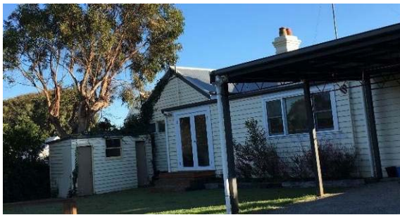
Rear of the house
