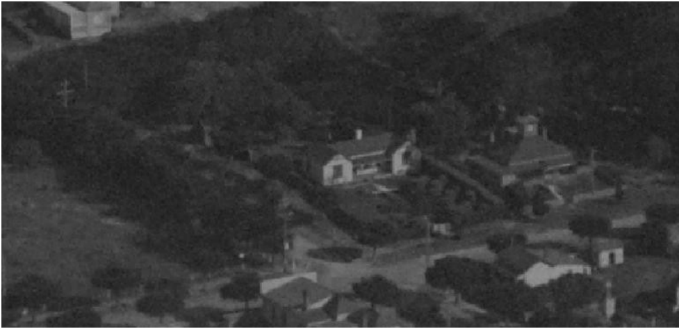
April 1936, prior to the alteration to the verandah. (Source: State Library of Victoria, H91.160/606)
