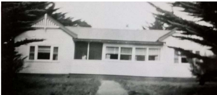
1955. Note the glass windows to the western part of the verandah. (Source: Thomas Family)
