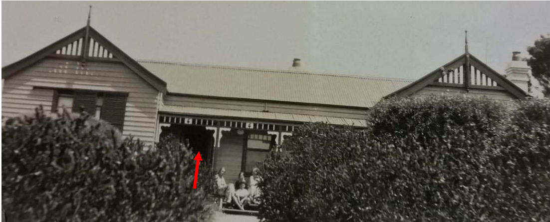
c.1930. The introduced gable end is on the left. The relocated entrance is indicated by an arrow. (Source: Thomas Family)
