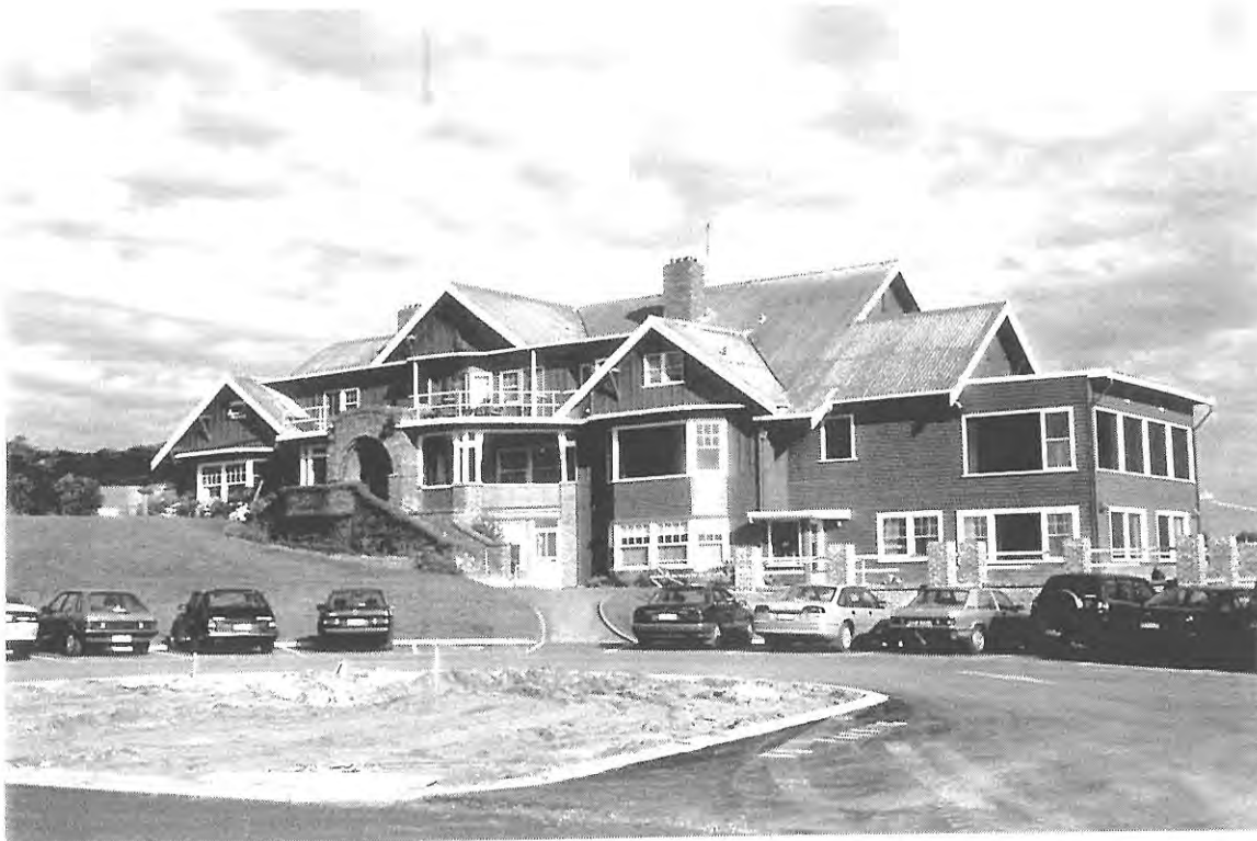
Figure 54 Barwon Heads Golf Clubhouse, Barwon Heads, 1920. Source: David Rowe, 1998.
