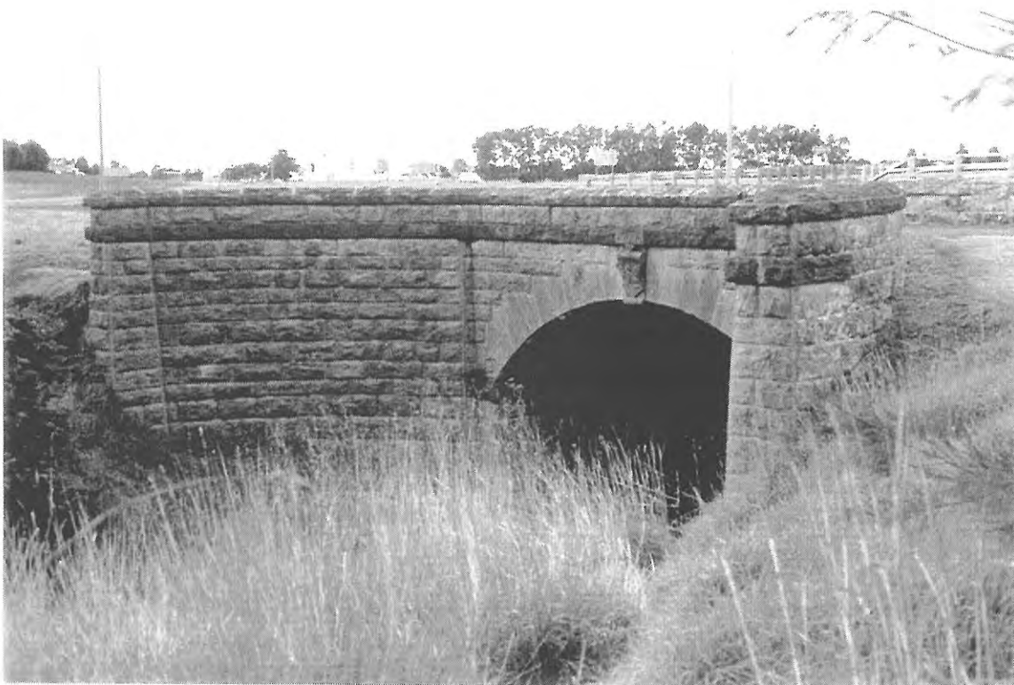
Figure 38 Road Bridge, Waurm Ponds, 1868. Source: David Rowe, 1998.
