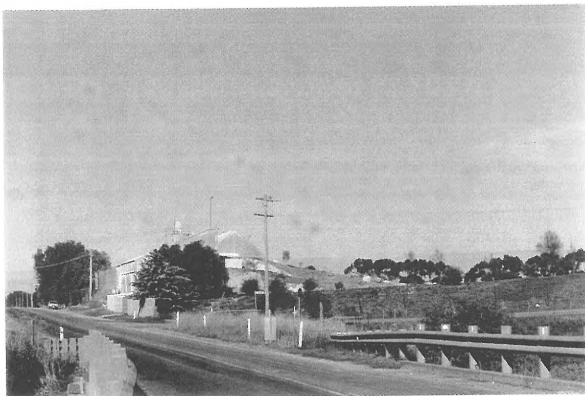
Figure 26 Lara Lime Company premises, Lara, 1862. Source: David Rowe, 1998.
