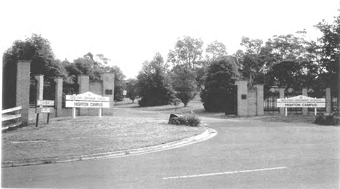
Figure 47 Geelong Grammar School Gates (formerly from The Hermitage), Waurn Ponds, 1963. Source: David Rowe, 1998.
