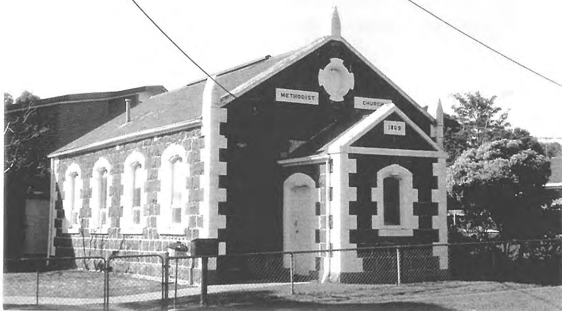
Figure 24 Methodist Church, Grovedale, 1869. Source: David Rowe, 1998.
