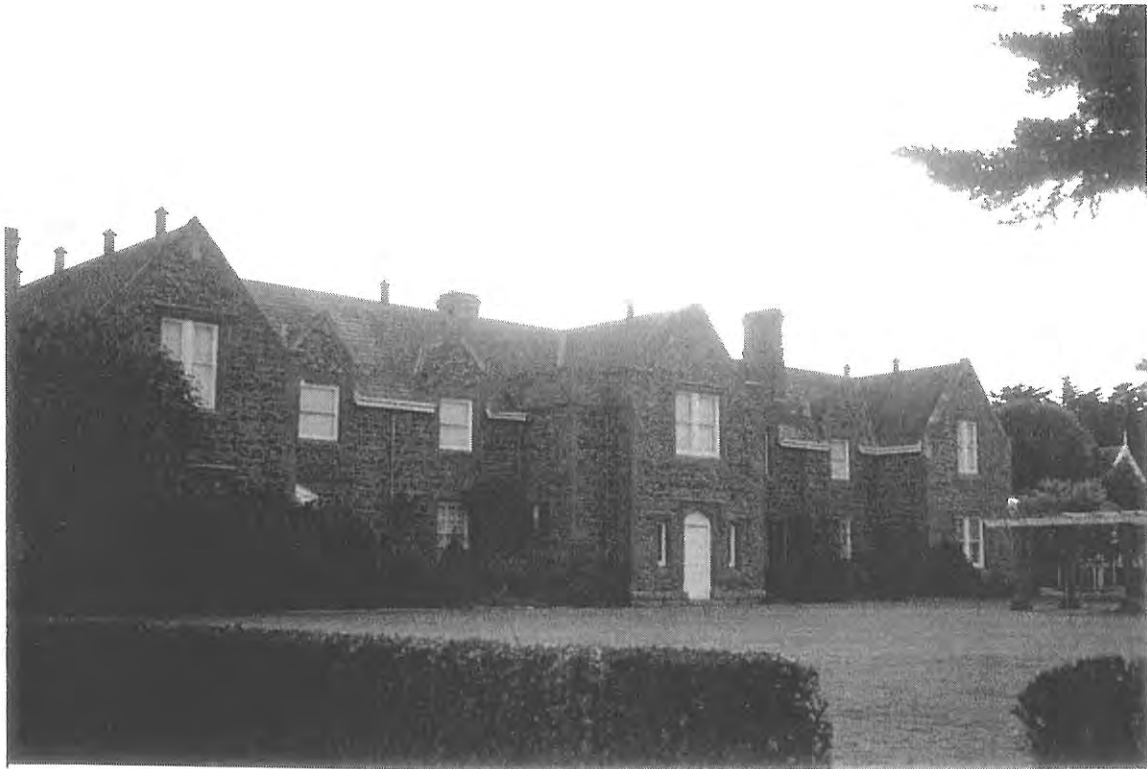
Figure 52 Geelong Cement Building (formerly Protestant Orphanage & School), Fyansford, 1855. Source: David Rowe, 1998.
