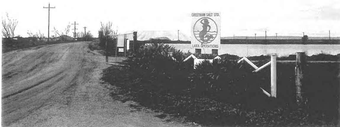
Figure 35 Cheetham Salt Works, Avalon, 1951. Source: David Rowe, 1998.
