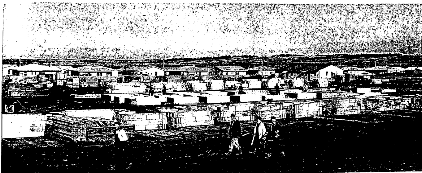
Figure 8 Workers and building components, Norlane Estate, 1953.
