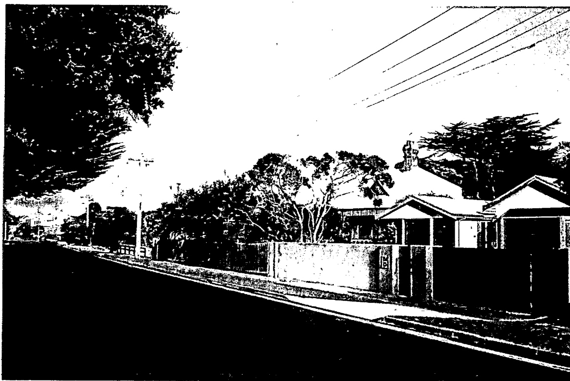
Flinders Parade, north end, view south. Detail of Monomeeth (left of infill house), with early and substantial cypress tree behind.
