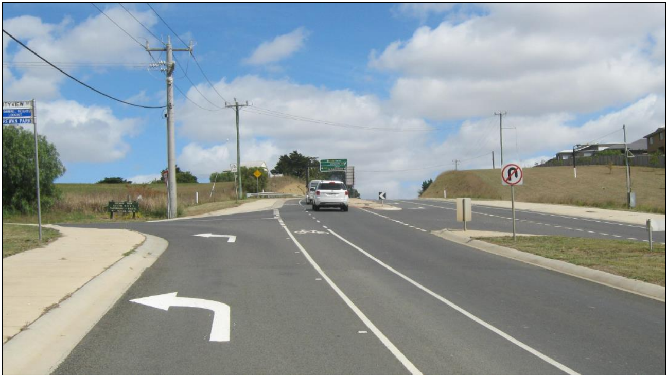
Figure 2-3 Barrabool Road looking west adjacent to the subject site
