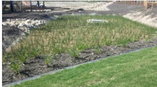
Figure 16: Typical biobasin constructed by Biofilta
