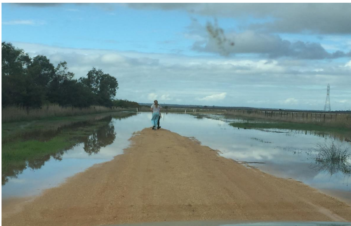
Figure 3 Flooding at Harriott Road 7
