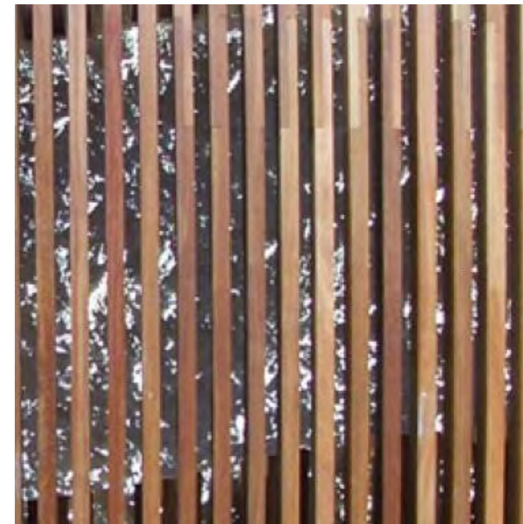
8 SEMI-TRANSPARENT TIMBER BATTEN CLADDING WITH GLASS BACKING (TO FRONT GATE + GARAGE PANEL LIFT DOOR)
