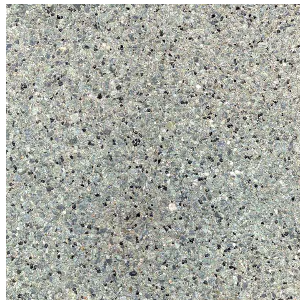
11 EXPOSED AGGREGATE DRIVEWAY
