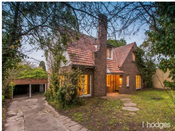
Front elevation of the former house (2015) (Source: Hodges website)
