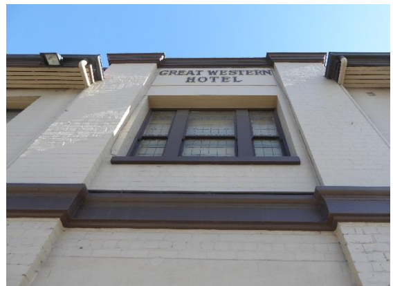
East elevation/Shannon Avenue, central bay
