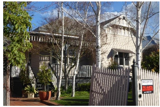
Federation period house, 16 Stephen Street
