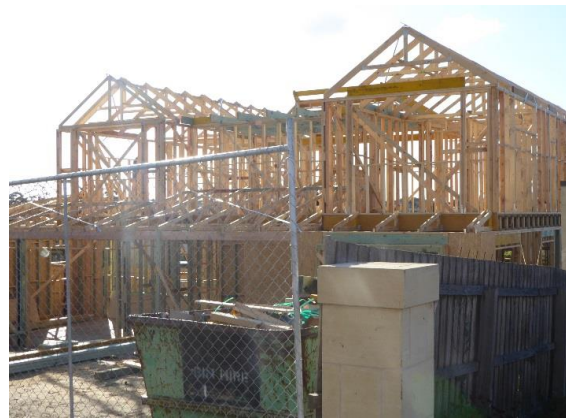
House under-construction, 25 July 2017
