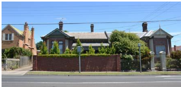
321-323 Shannon Avenue (Source: Newtown West Heritage Review, vol 1, NW04, April 2016, p1)
