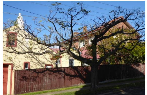
West elevation (Ruthven Street), garage (left) and house (right)
