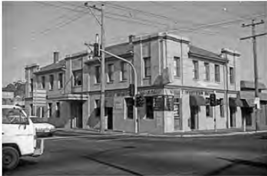
Figure 6: Great Western Hotel, east and north facades, 1994.
