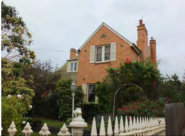
Photo 2: Front (east) elevation (from north side), 325 Shannon Avenue, May 2016.
