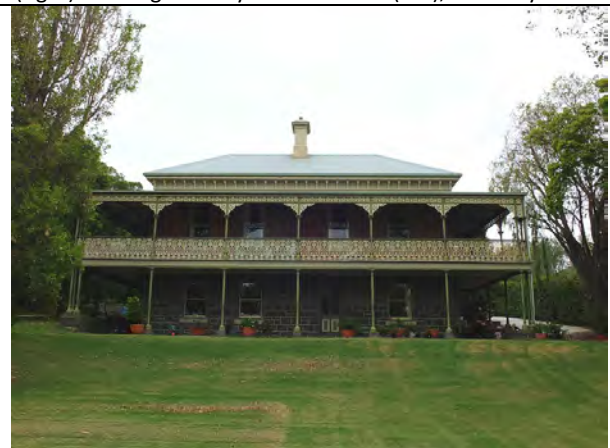
Photo 5: 'Newtown Brae', two storey addition built in 1885, March 2014.
