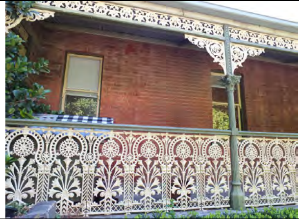
Photo 3: 'Newtown Brae', detail of east elevation showing delineation in the brickwork (centre) of the original dwelling (right) and single storey front addition (left), February 2016.
