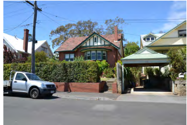
Photo 22: Dwelling, 16 Nantes Street, November 2015.
