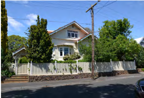
Photo 21: Dwelling, 12 Nantes Street, November 2015.
