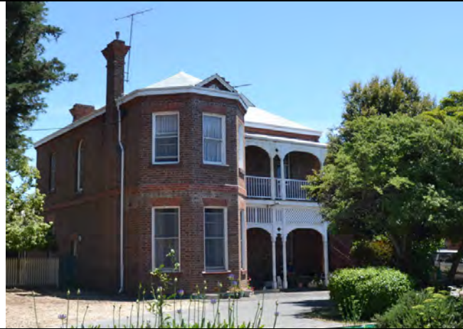
Photo 6: 'Brooklyn', principal (east) elevation, November 2015.
