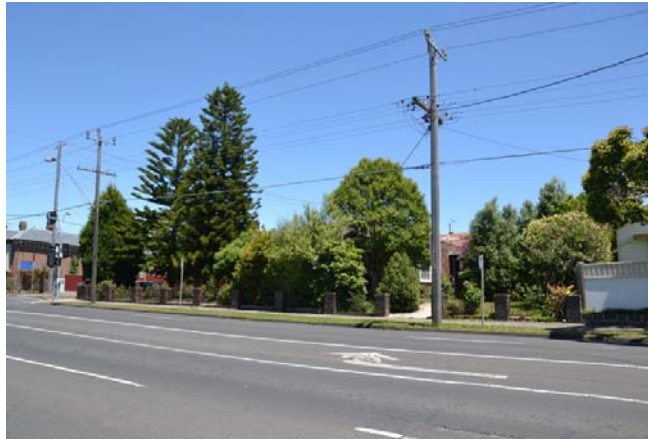
Photo 17: 319 Shannon Avenue, November 2015, showing early low, front fence with brick piers and plinth and open metal bays.
