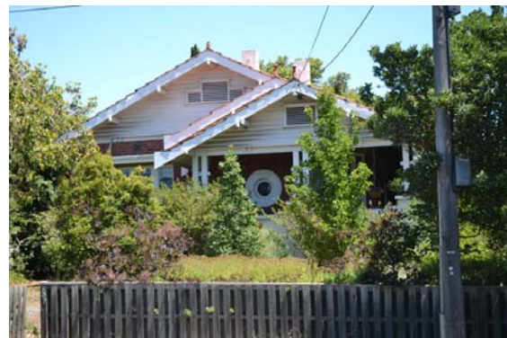
Photo 7: 'Banchory', 307 Shannon Avenue, November 2015.
