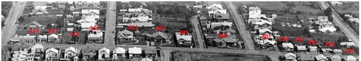
Figure 9: West Melbourne Road, showing properties on west side between 291 and 319 Shannon Avenue (with red numbers represent the current addresses of the properties), October 1927. Source: C. Pratt, La Trobe Picture collection, State Library of Victoria, accession H91.160/911.
