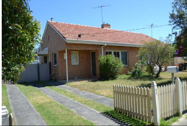
Photo 3: G.1 type semi-detached dwellings, 35-37 Churchill Avenue, November 2015.
