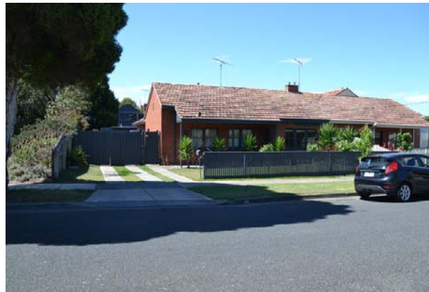
Photo 6: G.3a type semi-detached dwellings, 12-14 Churchill Avenue, November 2015.
