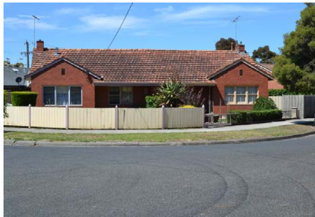
Photo 4: G.2 type semi-detached dwellings, 24-26 Churchill Avenue, November 2015.
