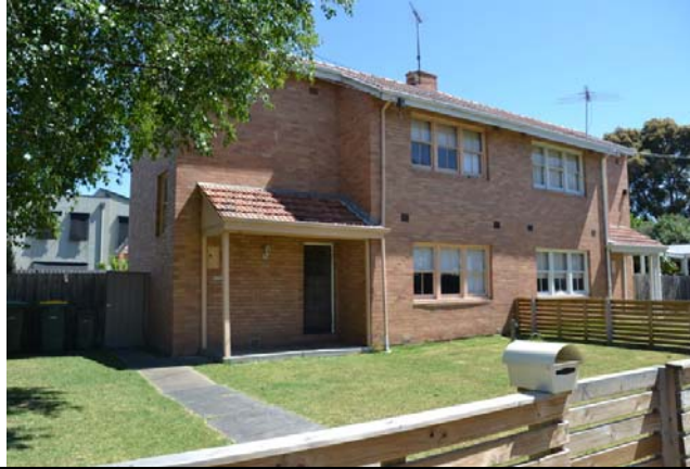
Photo 7: 2/G.3 type semi-detached dwellings, 23-25 Churchill Avenue, November 2015.
