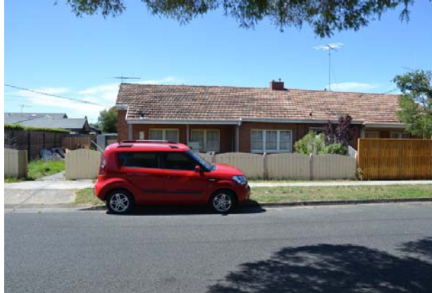
Photo 5: G.3 type semi-detached dwellings, 20-22 Churchill Avenue, November 2015.
