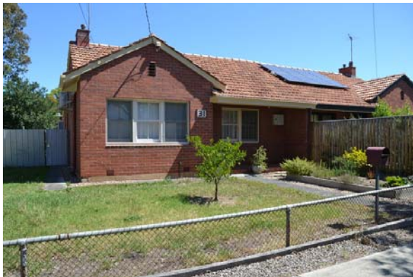
Photo 10: Original steel post & rail & chain mesh front fence, 31 Churchill Avenue, November 2015.
