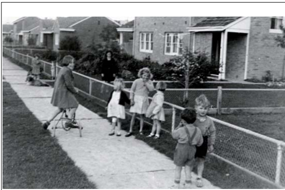
Churchill Avenue, 1945, with a portion of 25 Churchill Avenue in the foreground (right). Source: Department of Human Services online, February 2016.
