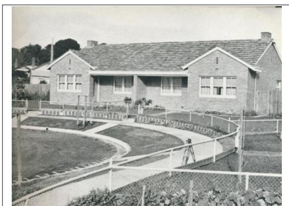
Duplex, 43-45 Churchill Avenue, 1942. Source: F. Oswald Barnett & W.O. Burt, Housing the Australian Nation, Ruckin Press at Victorian Places online http://www.victorianplaces.com.au/node/65381
