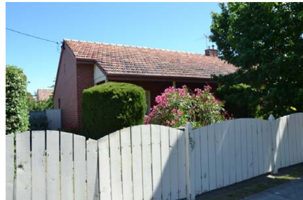
Photo 11: Introduced (early) front fence with expressed timber posts (having moulded cappings) and arched, wide timber picketed bays.
