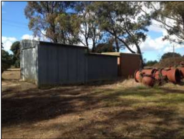
Plate 17: Maintenance sheds, looking south east
