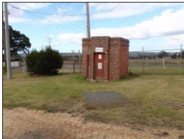
Plate 14: The 'Old meter Station' building adjacent the entrance gate on Thornhill Road, looking south
