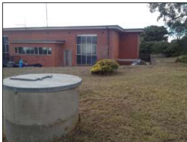
Plate 16: The pump station in the north west section of the study area, looking east
