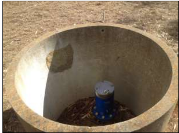
Plate 20: One of several concrete access pipes over the water pipe network
