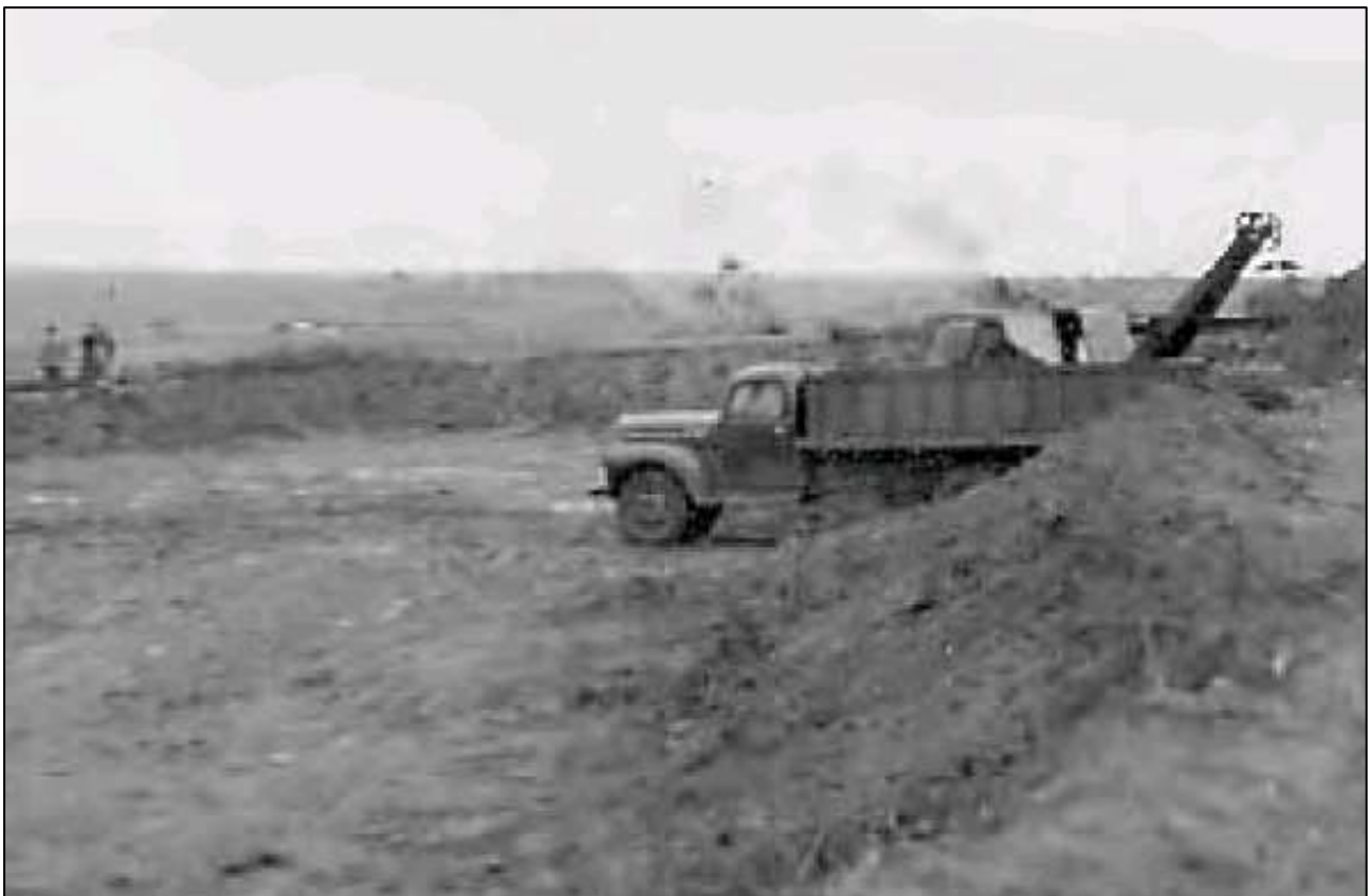
Figure 2: Excavaton of the Highton Basin during the late 1940s (Source: Edmonds 2005: 172)
