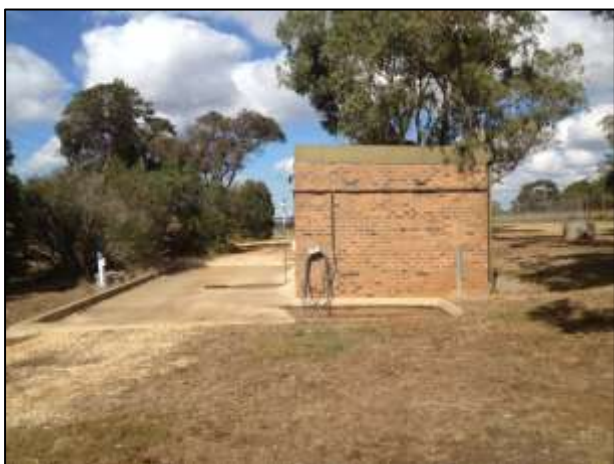
Plate 15: Disinfection Station and wash down area, looking south
