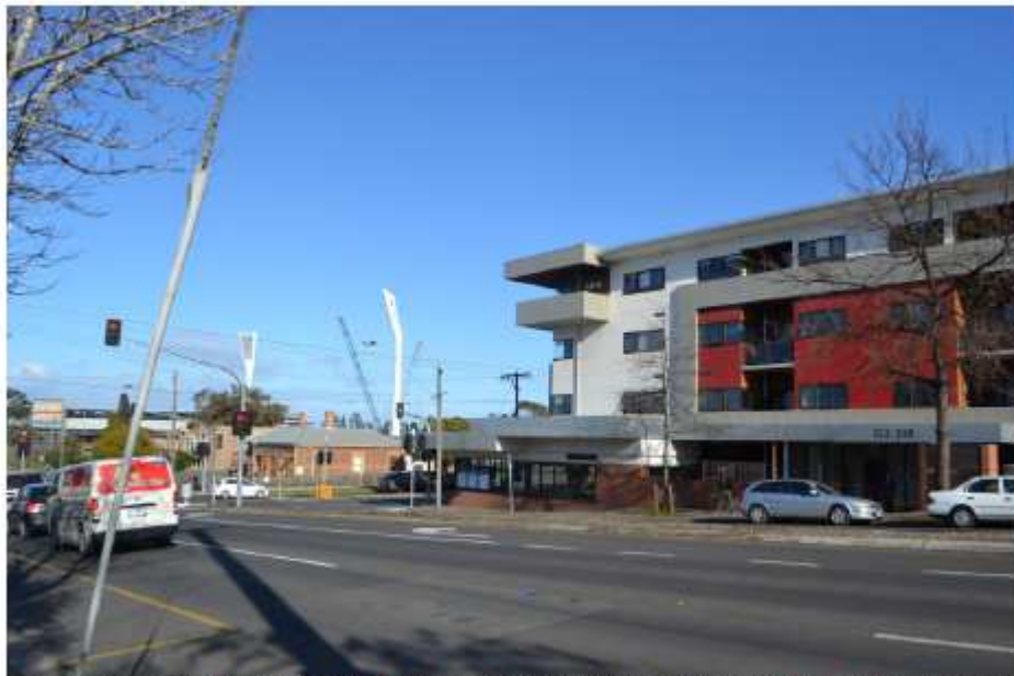
59 Kilgour Street visible in the bottom left corner of the apartment building, as seen from Moorabool Street.
