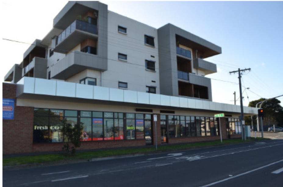
The three commercial tenancy's as seen from Kilgour Street at the ground level of the apartment building.
