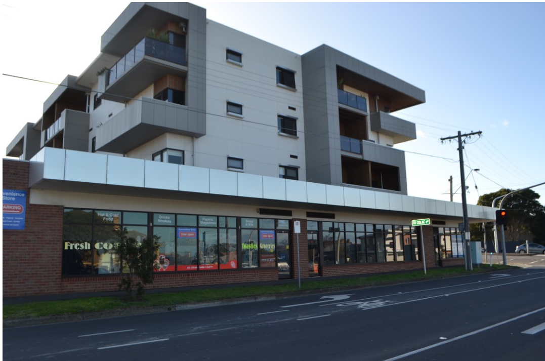
The three commercial tenancy's as seen from Kilgour Street at the ground level of the apartment building.
