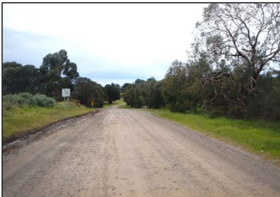
Figure 5: Gillies Road Looking South at the Drysdale Bypass Location
