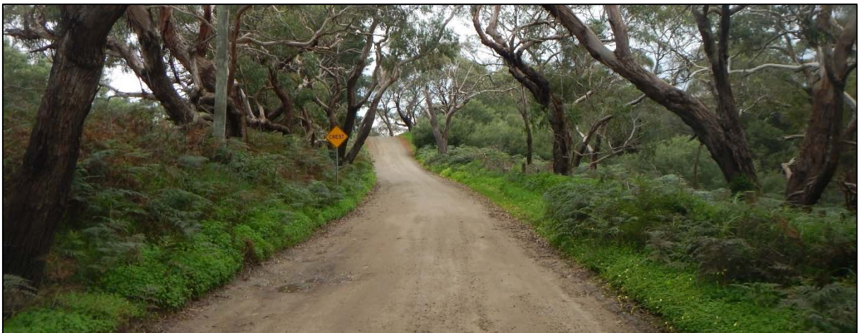
Figure 7: Basin Road Looking East
