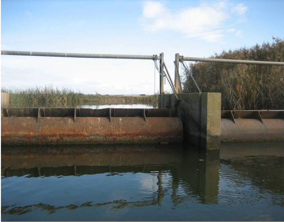
Figure 2 breakwater gates, prior to second gate being refurbishment
