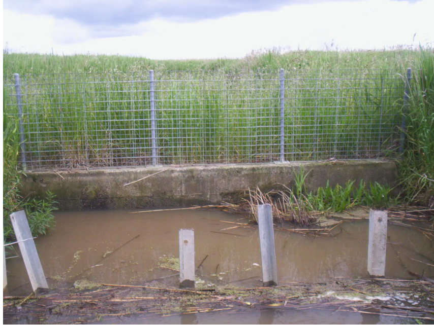
Figure 2-2 Reedy Lake Inlet Regulator Structure
